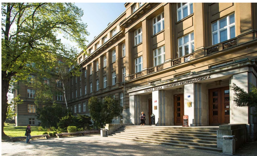
The entrance of the building B of University of chemical technology.
